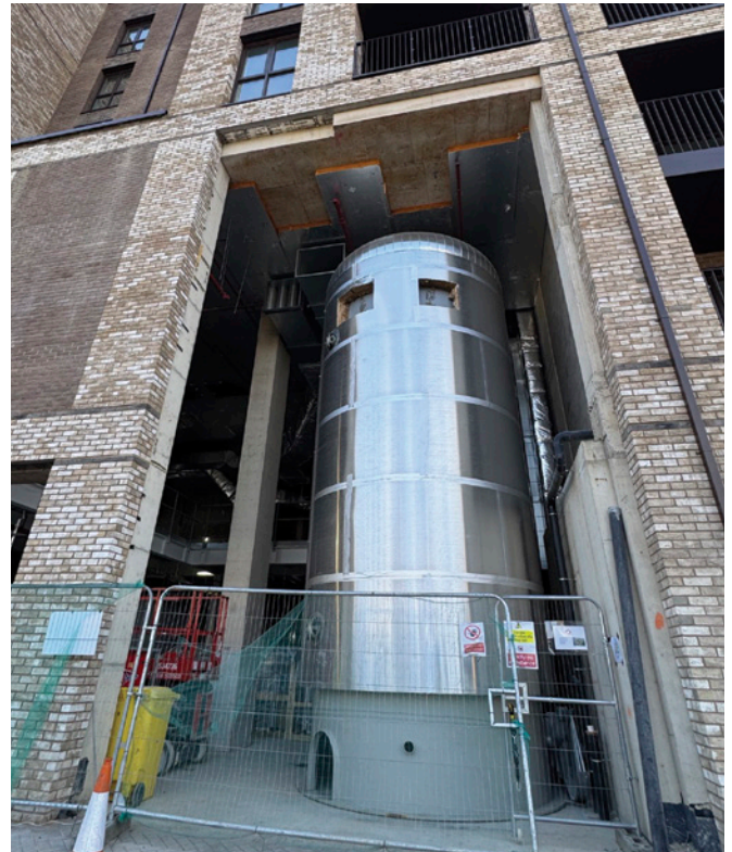
Clapham Park Energy Centre, hot water tank installation, 2024
